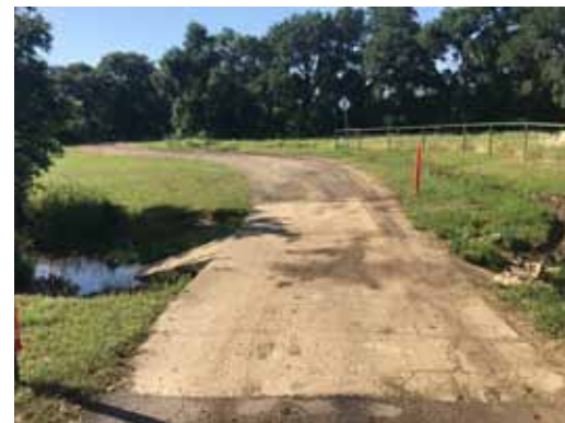
Exterior- Low Water Crossing
