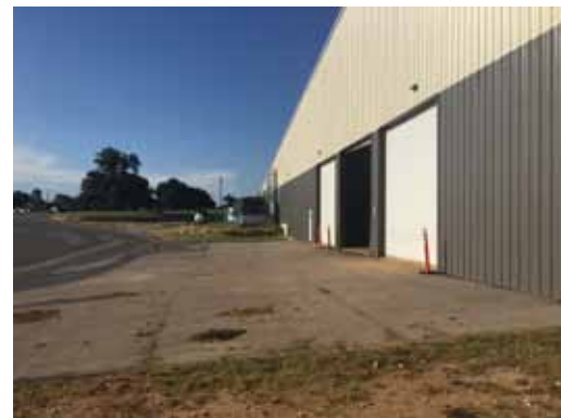
Event Center - East Entry to Staging Area
