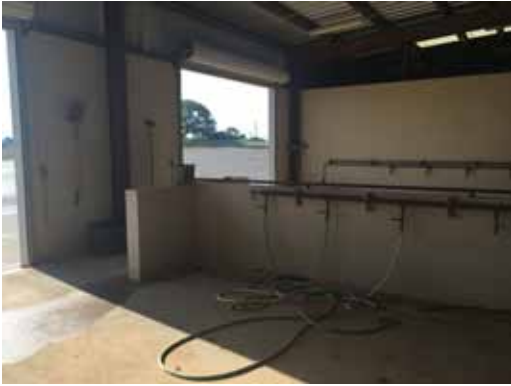
Event Center - Wash Down Area
