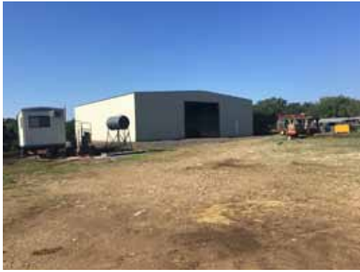
Exterior - Existing Barn - HCLE Owned
