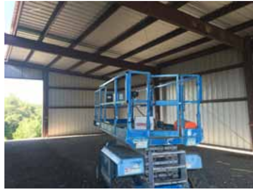
Exterior- Existing Barn (Interior) - HCLE Owned
