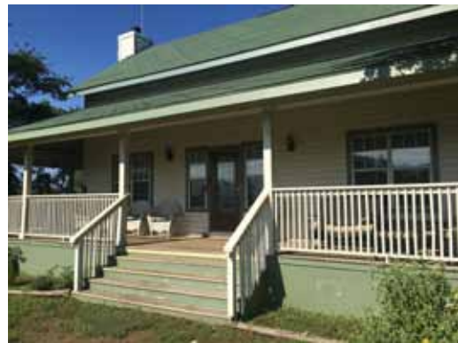
Exterior - Existing House
