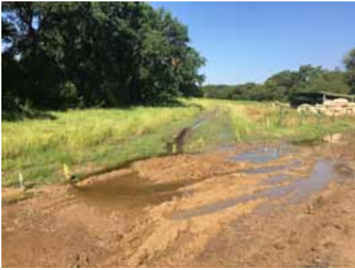
Exterior - Drainage Issues at Park Road
