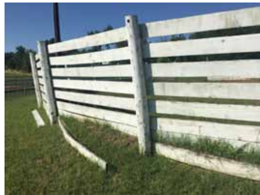
Exterior- Round Pen - Under Construction
