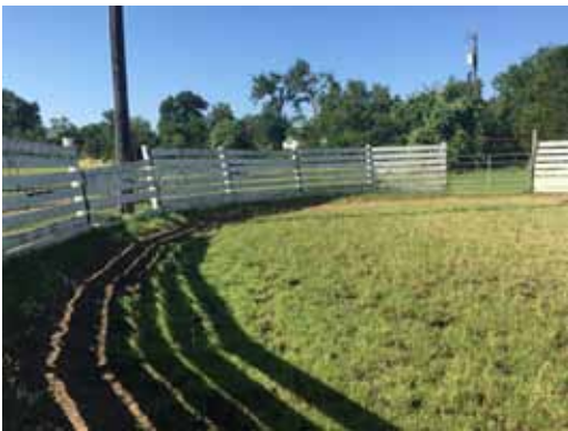
Exterior- Round Pen-Under Construction
